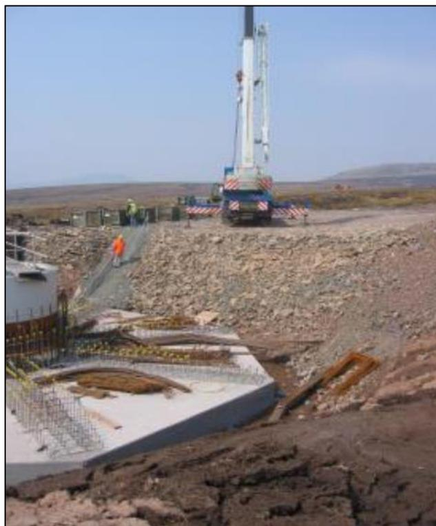
**Plate 6.1: Turbine foundation under construction with adjoining crane pad<sup>5</sup>**
