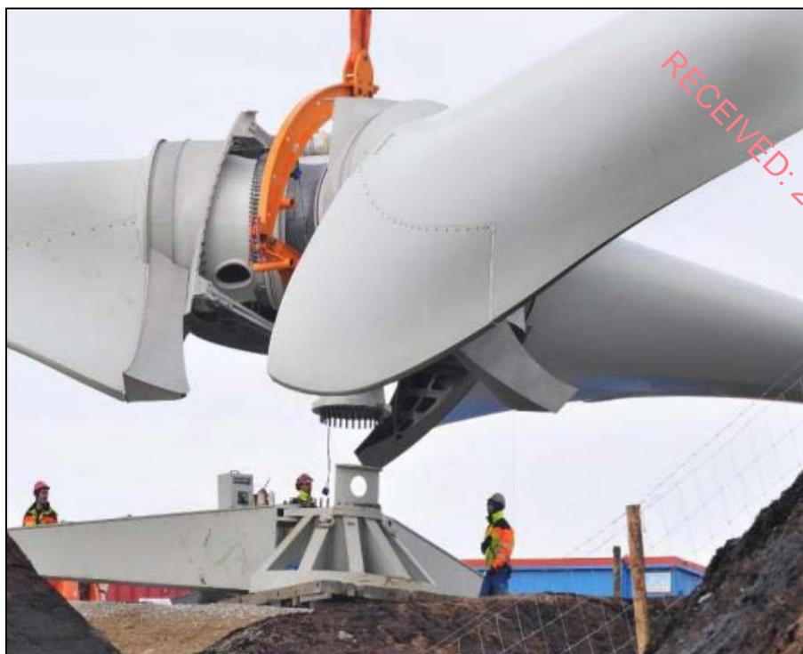
**Plate 6.4: Assembly of wind turbine blades <sup>2</sup>**
