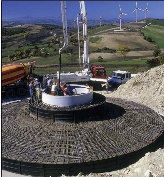
**Plate 6.2: Wind turbine foundation<sup>6</sup>**
