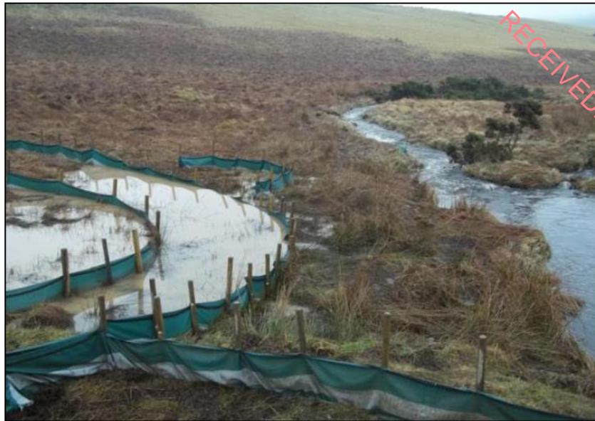
**Plate 1: Photograph of Silt Fencing**
